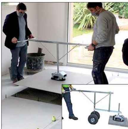
FXAH-120-GRABO-GREENLINE with FXAH-120-DUO-Set, bottom right: additionally with wheel set VPH-RS
