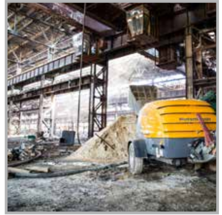
Russia, Ryazan placement of ~ 100,000 m 2 of screed
